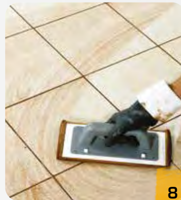
8 Complete the cleaning with a damp soft sponge, cleaning it frequently with a good amount of water.
