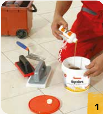
1 Pour all the catalyst (component B) into the paste (component A).
