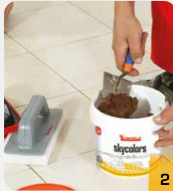
2 Mix the two components with a spatula.
