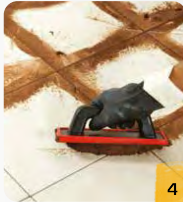
4 Apply the epoxy grout with a rubber trowel.
